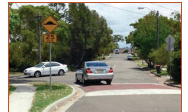
Transportation - Traffic Calming Raised Intersection Green (3) ..... Red (3) .....
